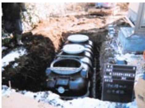
浄化槽設置の様相
